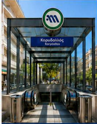
KORYDALLOS METRO STATION
